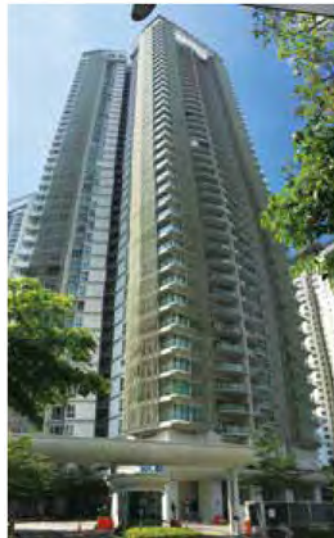
Project Name: MK28 Project Location: Kuala Lumpur , Malaysia
