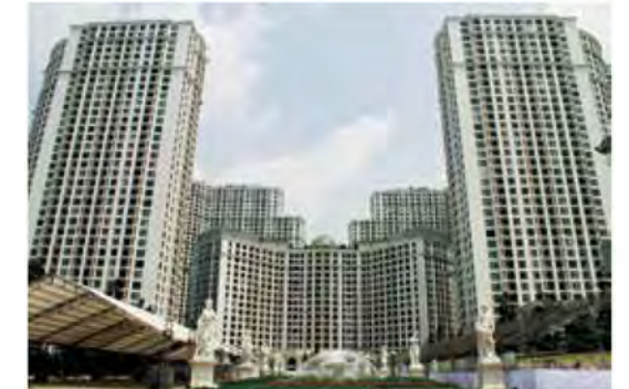
Project Name: Royal city Project location: Hanoi, Viet Nam
