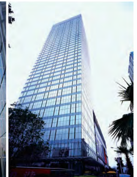
Glass Curtain Wall
