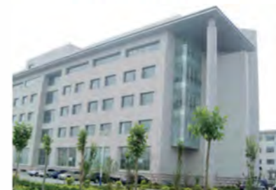
Stone Curtain wall
