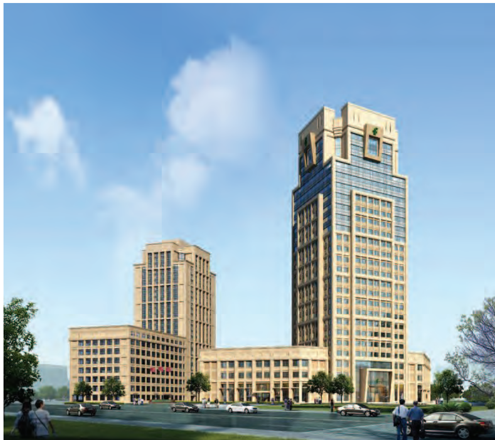
Postal Savings Bank of China
